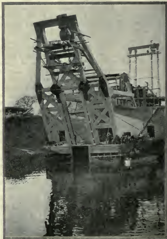
NATOMAS No. 8, DURING CONSTRUCTION.
